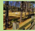
**91%** of the stormwater from the parking areas is filtered by plants and soils in a bioretention basin. This improves the quality of the groundwater, surface water, the landscape and helps protect the
