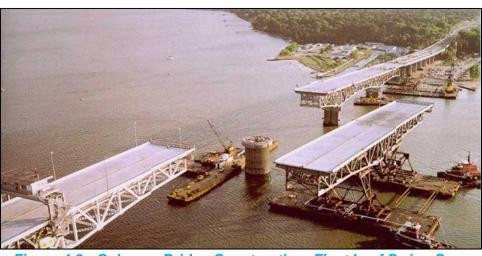
Figure 4-2: Coleman Bridge Construction: Float In of Swing Span
