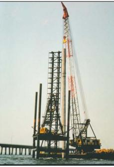
Figure 6-9: 66-inch Dia. Concrete Cylinder Pile Construction (Chesapeake Bay Bridge Tunnel Project)
