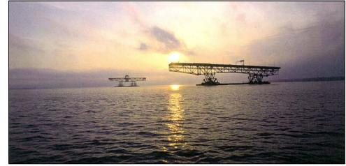
Figure 4-4: Coleman Bridge: Anchor span and Swing Span Afloat Awaiting Installation
