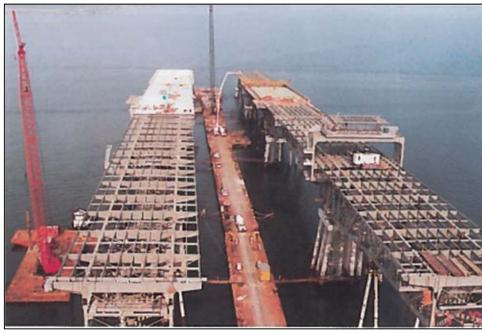
Figure 4-3: Coleman Bridge: Construction of Bridge in Fabrication Yard
