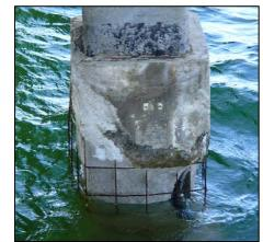
The approach and channel span units are supported on two-column piers with a partial height pier wall and some with pier caps, all founded on sunken caissons. These bents have isolated moderately sized spalls with exposed reinforcement but are generally in good condition. The structural adequacy of the approach and channel span piers is discussed further in Section 3.2.
