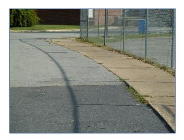
**Figure 4.** The sidewalk along Bessie Weller Drive is level with the roadway at points.
