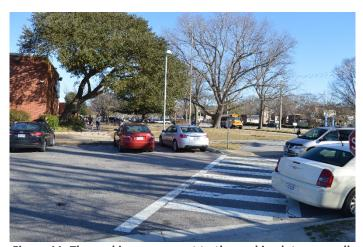
Figure 11: The parking space next to the parking lot crosswalk is situated in such a way that drivers using this space must back up into the parking lot crosswalk.
