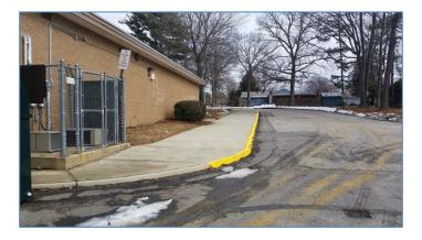
**Figure 8. School property at Ashwood Road (facing east).** There are no marked crosswalks or curb ramps at this intersection.
