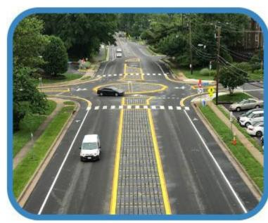
Figure 13 Modular temporary roundabout in Fairfax County
