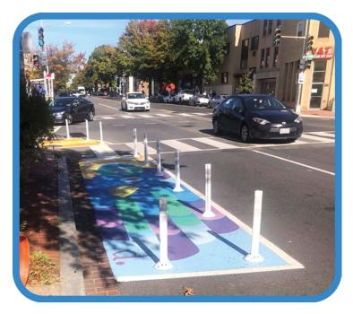
Figure 12. Flex-post curb extensions with paint at a crosswalk in Washington, DC.
