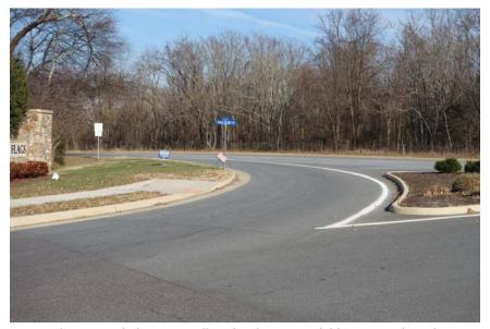
Figure 19: Missing crosswalk and curb ramp at Field Stone Boulevard
