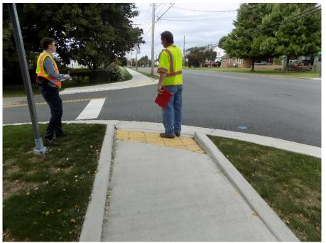
Figure 25: New Sidewalks and Curb Ramps along Stuart Avenue (US 340) at C Street
