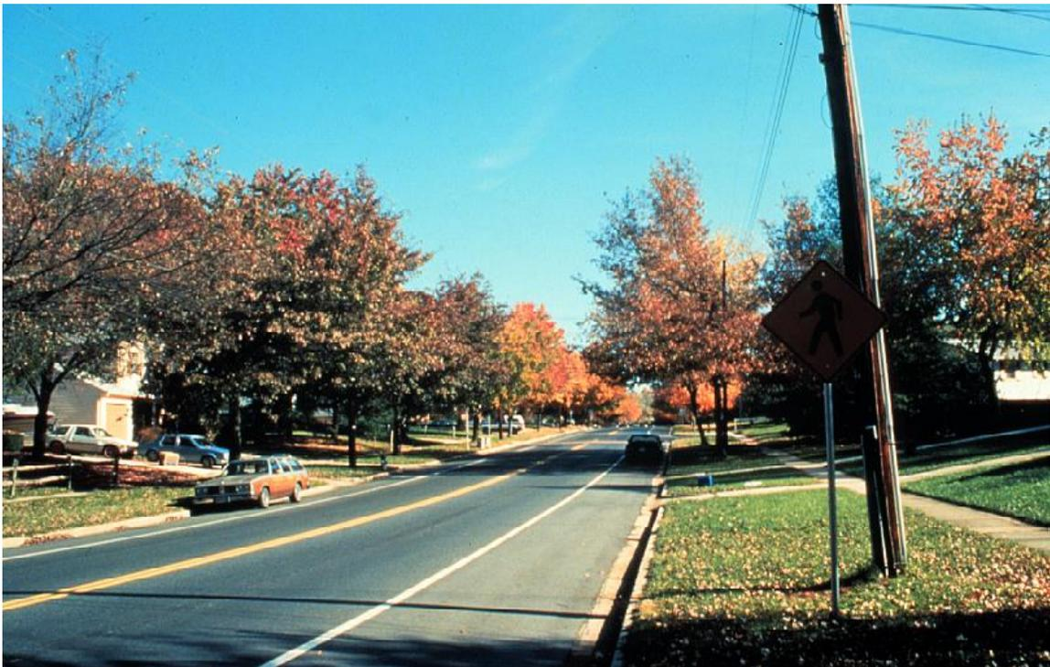
**Figure 2.4 – Narrow travelway by re-stripping pavement for a bike lane**
