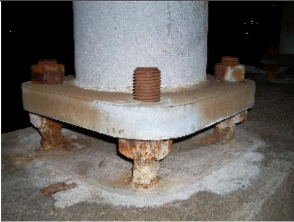
Rusted anchor bolts and missing nut
