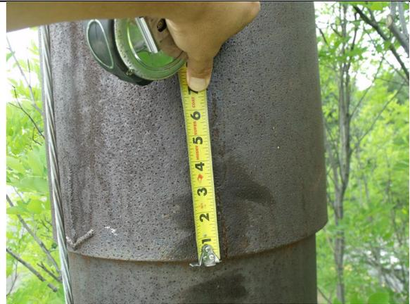
4" vertical crack at the slip joint
