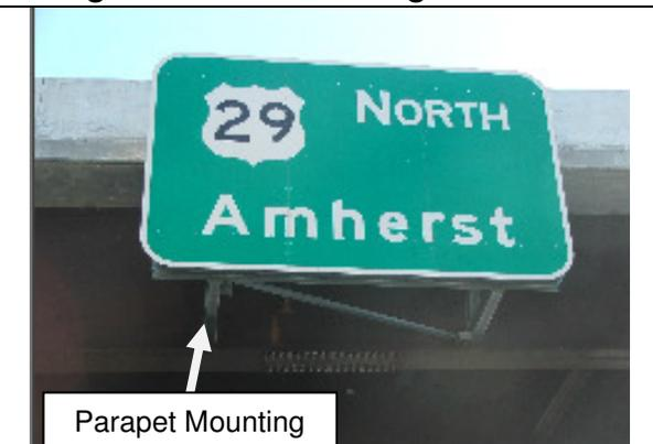
Figure 4 – Parapet Mount Sign Structure
