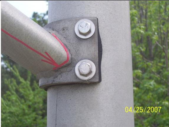
Lower arm of luminaire chord has a 3.5" fatigue crack in weld at connection to pole
