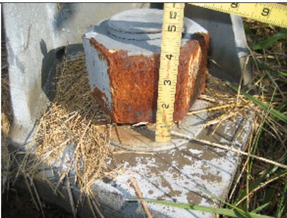
Loose anchor bolt with 1" gap between nut and base plate
