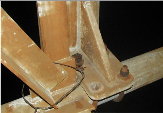
U-bolt sheared at left front pole to bottom chord Connection
