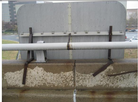
Twisted anchor clamp over the parapet
