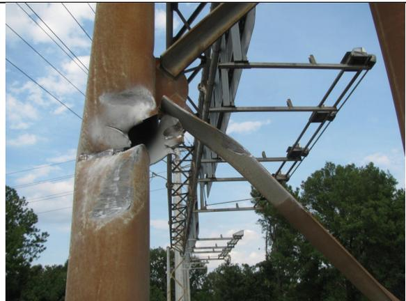
Column torn and bent 3" at point of impact
