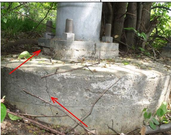
Deteriorated grout pad and cracked pedestal
