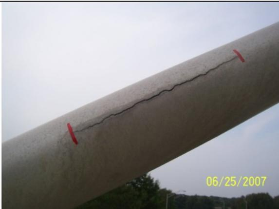
6" crack in lower chord of luminaire
