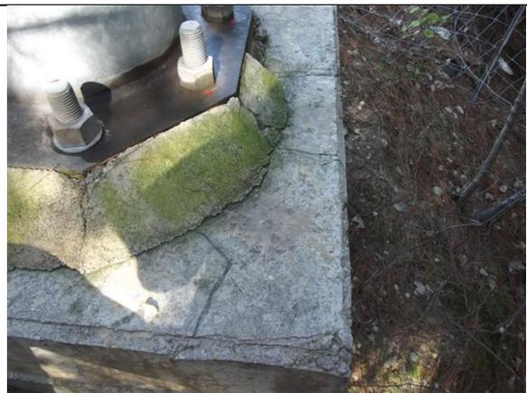
Deteriorated and cracked grout
