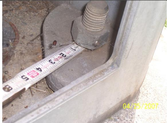
Loose anchor bolt nut at luminaire base
