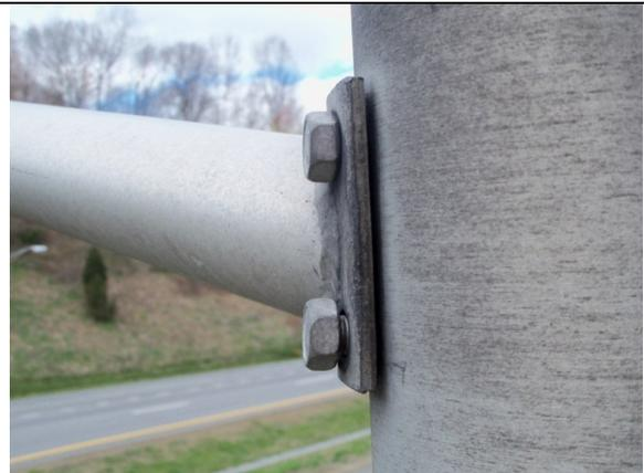
Two of four bolts loose in top chord connection to luminaire pole
