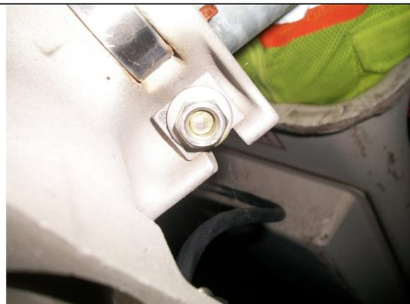
Nut on strap bolt for signal from pole lacks 50% thread contact
