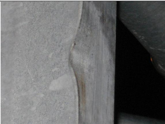
Damaged & bent flange of vertical hanger
