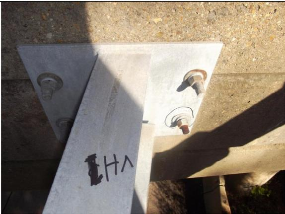
Failed mounting bolt (circled)
