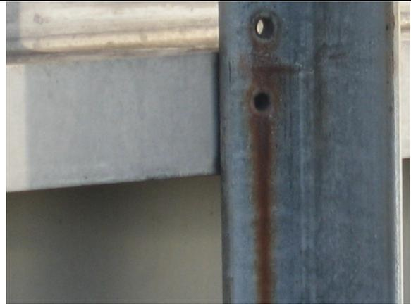
Missing bolt at wind beam to vertical hanger connection
