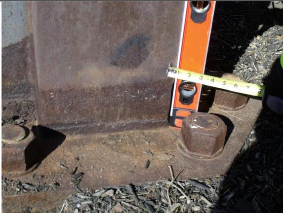
Section loss to the bottom of the pole.
