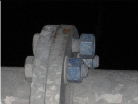
Loose Bolt at splice plate.
