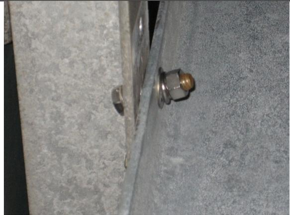
Poor vertical hanger connection with the Z-bar
