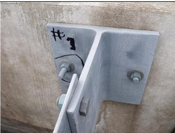
Failed bolt (circled) at parapet mount.
