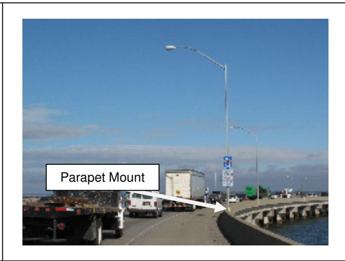
**Figure 6 – Parapet Mounted Luminaire Structure**
