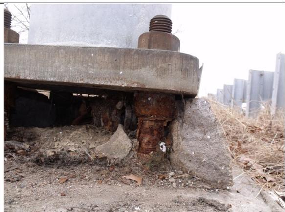
Severely corroded anchor bolts exposed when grout has fallen away
