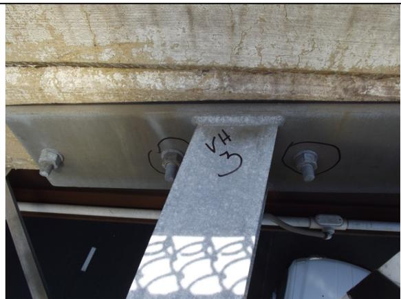
Two failed bolts (circled) at parapet mount
