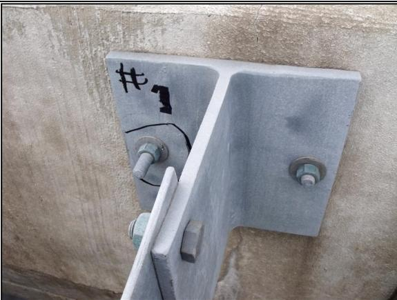
Failed bolt (circled) at parapet mount.
