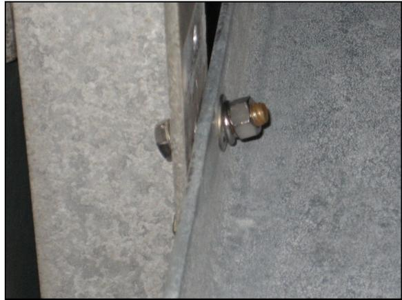
Poor vertical hanger connection with the Z-bar
