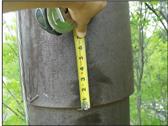
4" vertical crack at the slip joint
