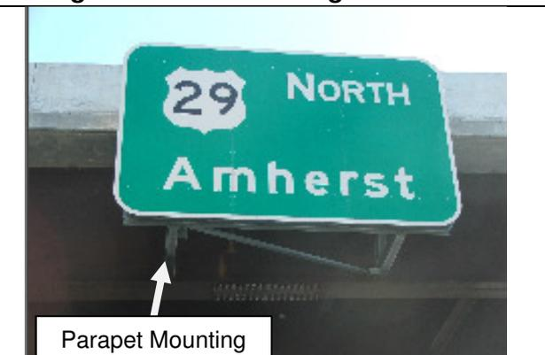
**Figure 4 – Parapet Mount Sign Structure**
