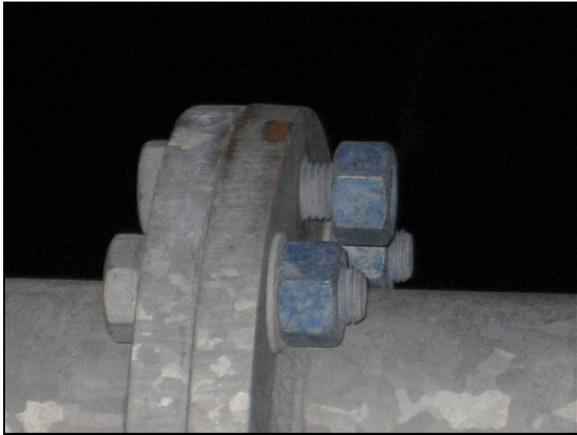
Loose Bolt at splice plate.
