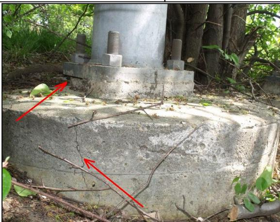
Deteriorated grout pad and cracked pedestal
