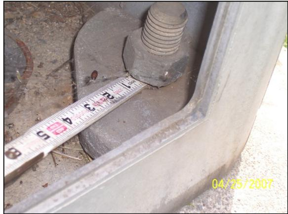
Loose anchor bolt nut at luminaire base
