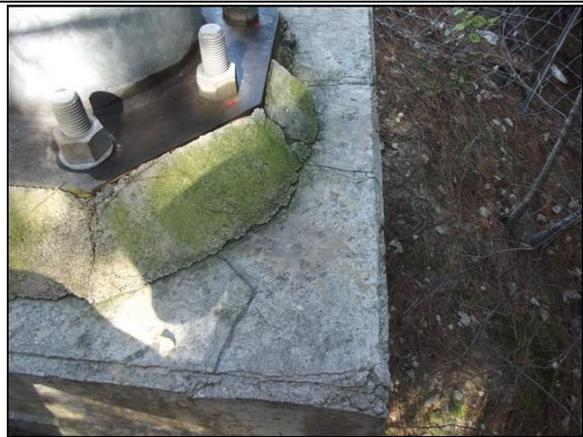
Deteriorated and cracked grout
