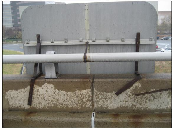
Twisted anchor clamp over the parapet
