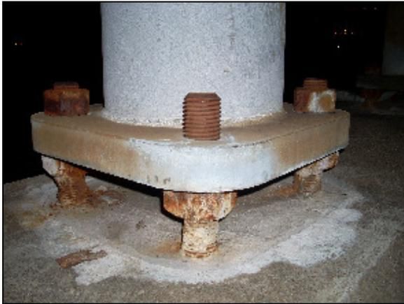
Rusted anchor bolts and missing nut
