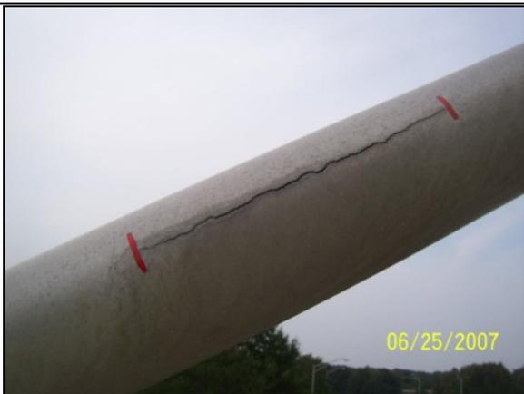
6" crack in lower chord of luminaire
