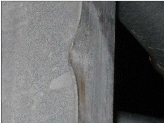
Damaged & bent flange of vertical hanger
