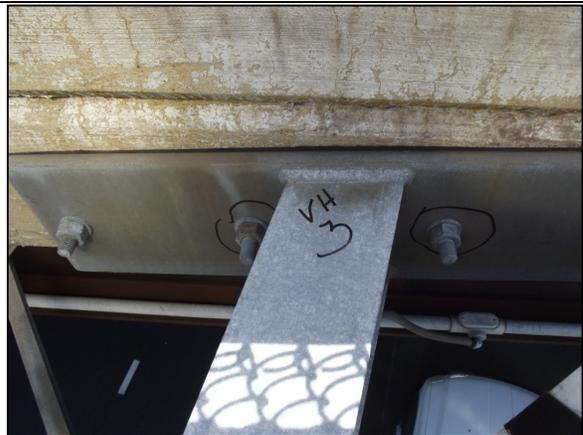
Two failed bolts (circled) at parapet mount
