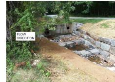
CONCRETE HEADWALL WITH 18" & 36" RCP OUTLETS
