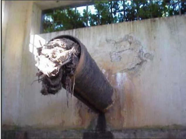
Any trash or debris that is blocking or impeding operation of an outflow structure shall be removed so that the outflow is fully functional again. Inspect the condition of overflow pipes, the overflow filter path and/or secondary runoff reduction practices. This trash or debris, either “natural or “man-made,” shall be disposed of in accordance with the waste classification and hazard level.
