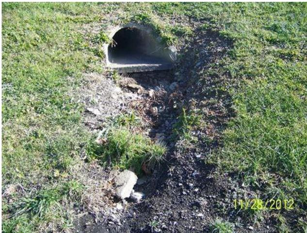
Outlet protection shall be repaired/installed per the original approved plans, including include riprap footprint dimensions, size of stone and placement specifications. If the original design plans are not available or if the original design is clearly inadequate, which is evident by the presence of erosion and scour, the outlet protection shall be designed by a qualified VDOT representative or employee and repaired in accordance with the applicable specifications and design requirements.
