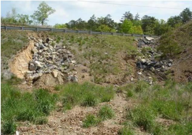
Outlet protection shall be installed per the original approved plans including the dimensions, size of stone and placement specifications. If the original design plans are not available or if the original design is clearly inadequate, the outlet protection shall be designed by a qualified professional in accordance with the applicable specifications and design requirements. All outlet protection shall be installed per the approved E&S Annual Standards and Specifications.
