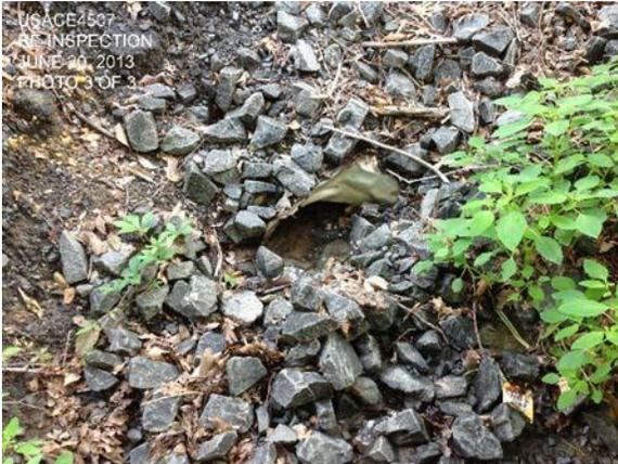
Any trash or debris that is blocking or impeding operation of an outflow structure shall be removed so that the outflow is fully functional again. This trash or debris, either “natural or “man-made”, shall be disposed of in accordance with the waste classification and hazard level. Blockages have the potential to increase the water level in the facility beyond design levels.
