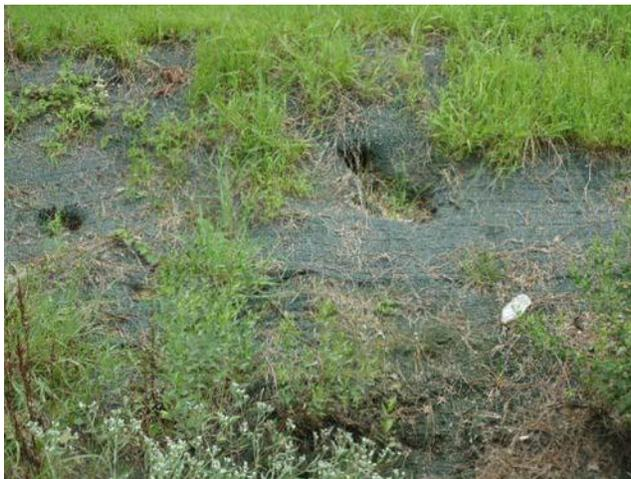
All animal burrows shall be filled and compacted. Attention should be given to ensure that the burrow has not affected the structural integrity of the infiltration facility. If the structural integrity is comprised, a qualified VDOT representative shall be contacted for further investigation to determine appropriate structural repair measures.
