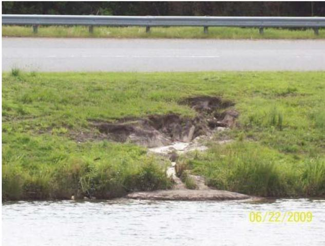
Both the upstream and the downstream side of all check dams shall be inspected for signs of undercutting and erosion. Erosion shall be corrected by seeding, grading, and/or installation of soil stabilization matting to correct the deficiency. If the erosion is compromising the BMP's structural stability, a competent VDOT representative shall be consulted to determine the proper repair and methodology, such as soil type and compaction requirements, to ensure structural stability of the facility.
