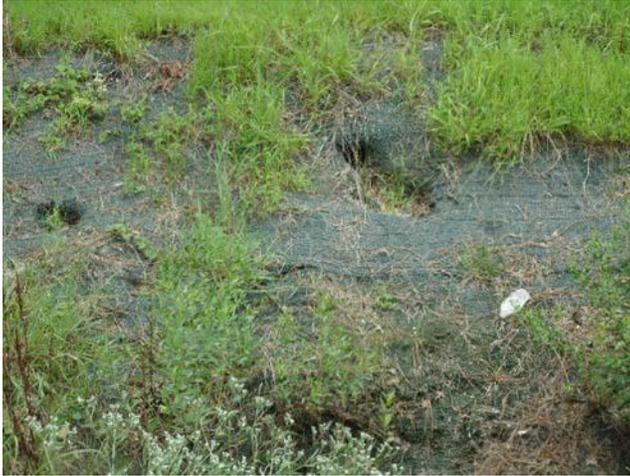
All animal burrows shall be filled and compacted. Attention shall be given to ensure that the burrow has not affected the structural integrity of the basin. If the structural integrity is comprised, an appropriate qualified VDOT representative shall be contacted for further investigation and to determine appropriate structural repair measures.
