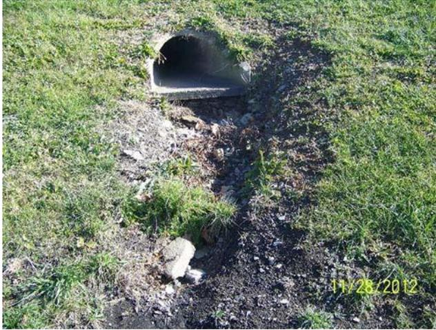
Outlet protection shall be installed per the original approved plans including the dimensions, size of stone and placement specifications. If the original design plans are not available or if the original design is clearly inadequate, the outlet protection shall be designed by a qualified professional in accordance with the applicable specifications and design requirements. All outlet protection shall be installed per the approved E&S Annual Standards and Specifications.
