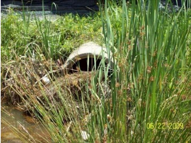
Any trash or debris that is blocking or impeding operation of an inflow structure and/or forebay shall be removed to restore proper function. This trash or debris (either “natural or “man-made”) shall be disposed of in accordance with the waste classification and hazard level.
