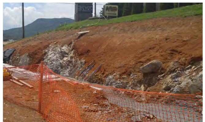
Variable depth to rock with limestone pinnacles, ledges, and cutters (soil slots) over relatively short distances at the VDOT I-81 Exit 150 project in the Salem District is typical of area conditions.
