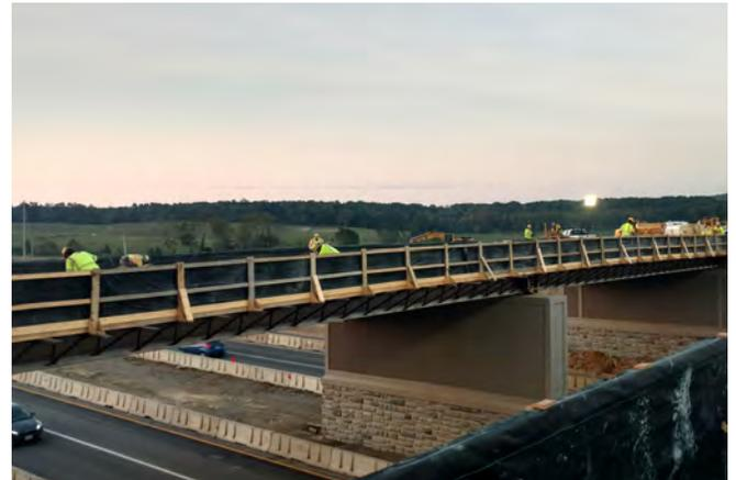
Construction QC team checking bridge deck prior to pour.
