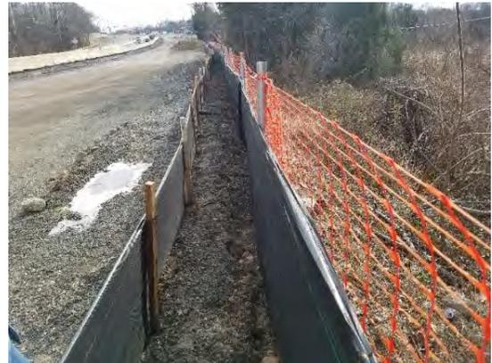
**Figure 4.4.1.2** - Installation of silt and safety fence to ensure avoidance of impacts to non-permitted areas, protected properties, and commitment areas.
