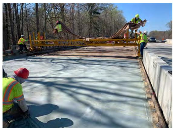
Figure 4.5.1.11 - Bridge Latex Modified Concrete Overlay
