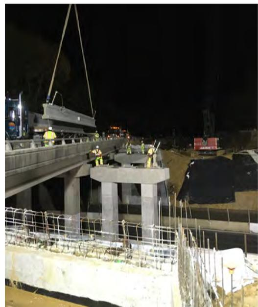
**Figure 4.5.3.2.8** - Beam Erection at Widened Bridges
