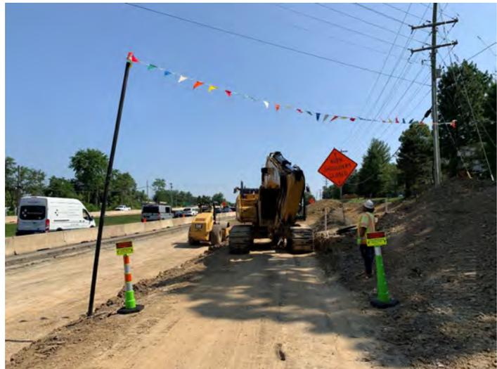
**Figure 4.4.2.2** - Overhead utility protection measures including low-clearance flagging, warning signs, and spotter.
