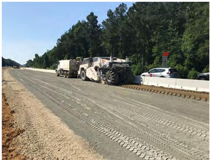
Figure 4.5.1.5 - Cement Treated Crushed Concrete Subbase Layer Option
