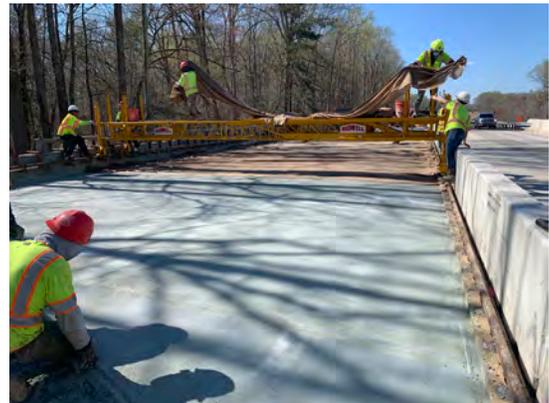
Figure 4.5.3.2.11 - Bridge Latex Modified Concrete Overlay
