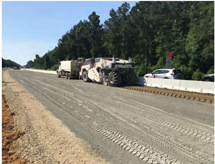
**Figure 4.5.3.2.5** - Cement Treated Crushed Concrete Subbase Layer Option
