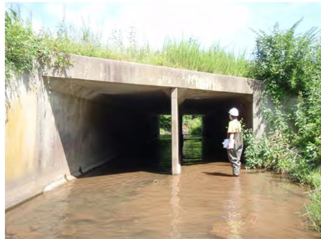
Figure 4.3.2.6 - Box culvert inspection.
