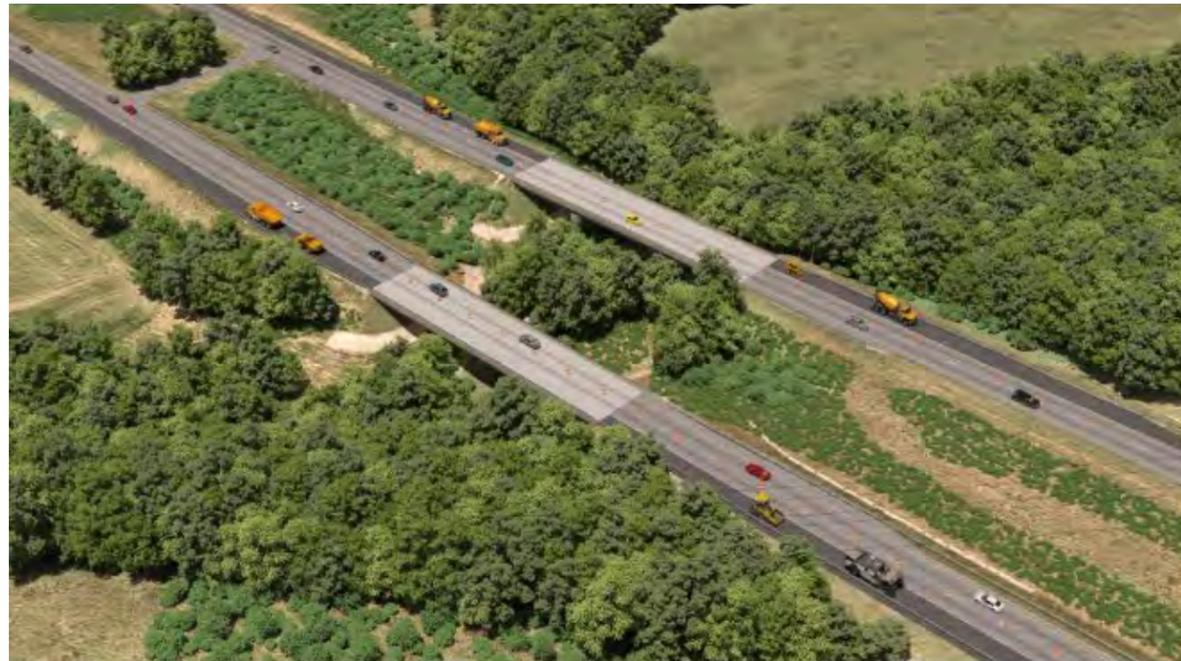
Roadway and bridges are one lane; no traffic shifts required between roadway and bridge
