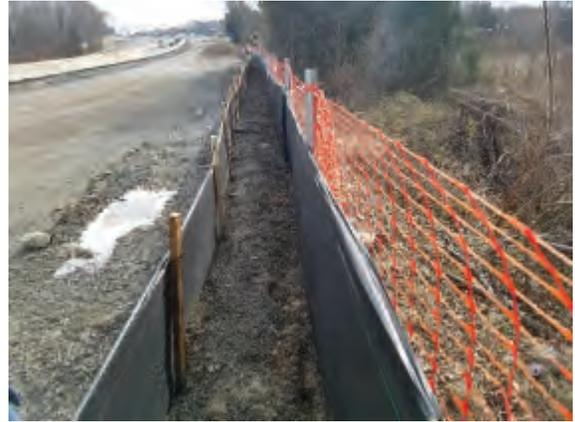
Figure 4.4.1.2 - Installation of safety fence to ensure avoidance of impacts to non-permitted jurisdictional areas.
