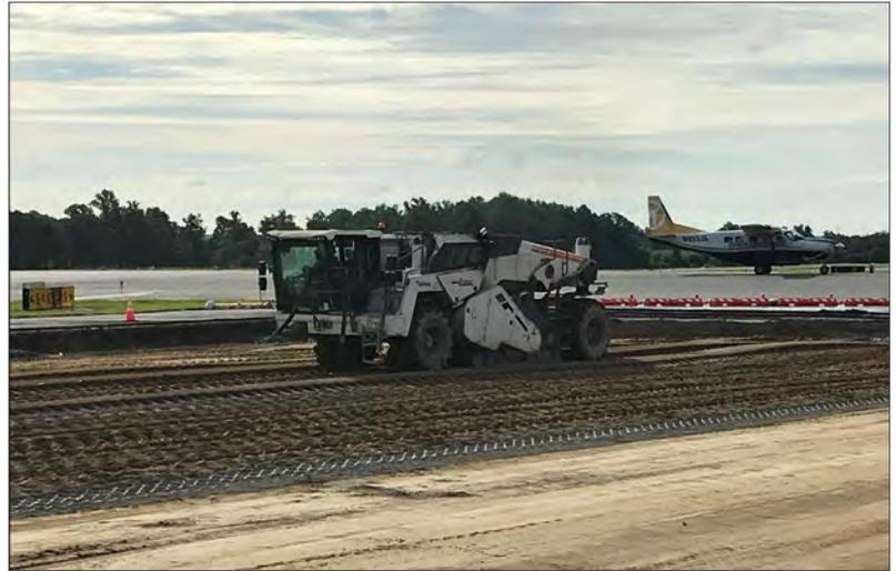
When we implement chemical modification of subgrade soils or improve ground stiffness with aggregate piers, our geotechnical designer will be onsite to confirm the design intent is being met. Design staff input will be used not only to confirm the ground is reacting to the treatment as anticipated in the design, but also to determine if a larger or smaller area requires treatment.
