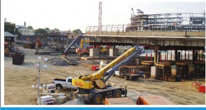
superstructure demolition will require nighttime I-64 traffic restrictions, including lane closures, since this work spans multiple travel lanes. Installed shielding will ensure that other GBB superstructure construction activities will have minimal impact on I-64 traffic. Demolition of the existing GBB abutments, end spans, and outer piers can coincide with the exterior roadway work in the second and third East 1 MOT phases.
