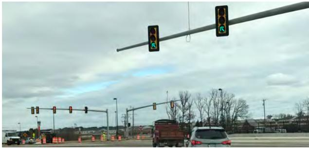
*Confusing signal head placement which can cause left turn movement traffic to stop at thru movement signal*
