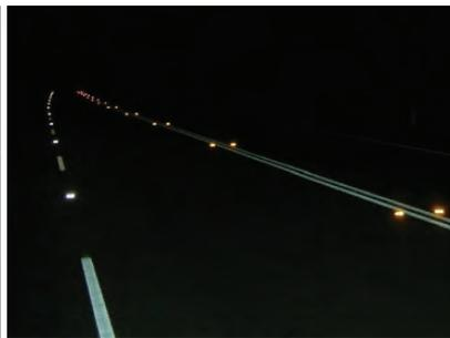
2. RPM reflectors enhance lane lines
