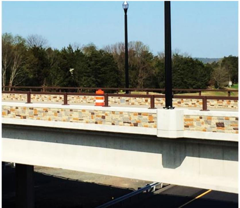
*Figure 4.3.2-4 Bridge Parapet with tri-colored Drystack Architectural Treatment: Example from Lane's I-66/Route 15 project.*
