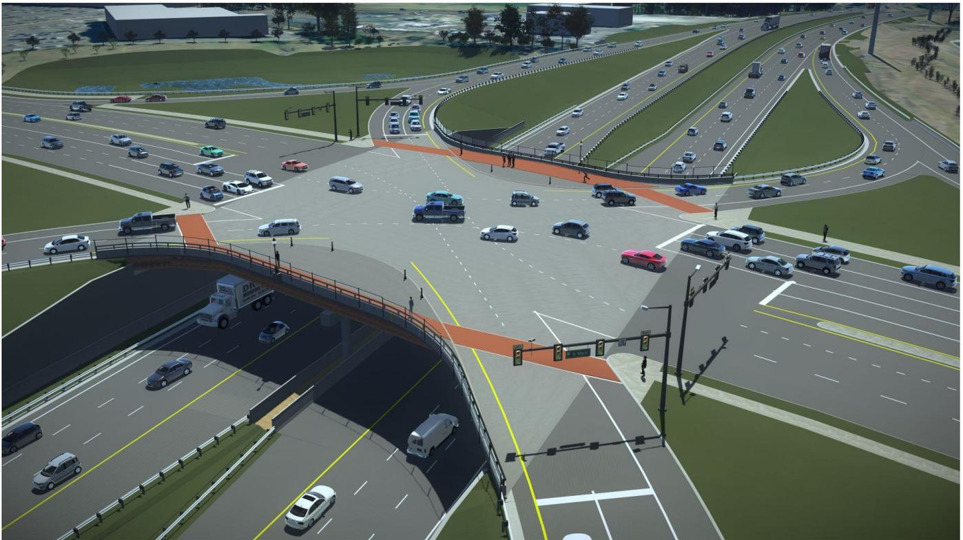
Figure 4.3.2-1: SPUI Bridge looking East (some details omitted for clarity)
