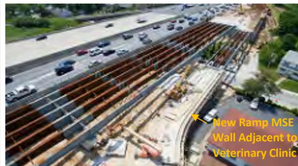
and the project-wide TMP. The TMP required consideration of impacts to bus routes, fire/rescue, truck traffic, and access to adjacent businesses. AMT's construction drawings depicted pavement construction, proposed realigned ramp, retaining wall and sound wall, improvements to sidewalks, and phased MOT plans. Storm water design included bioretention, extended detention, temporary erosion and sediment control plans, and storm drain plans/profiles.
