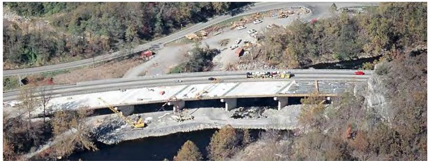
*Traffic shifted in a one-lane, two-way pattern, to allow demolition and construction to progress on Branch's I-64 Jackson River project.*
