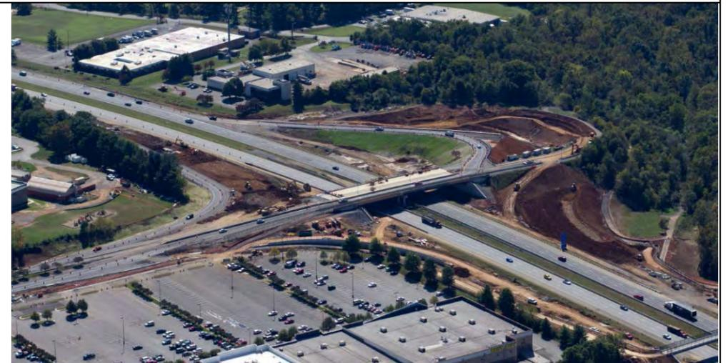
**Structures** | STV developed design plans for the widening and rehabilitation of the bridge carrying Valley View Boulevard over I-581, a shared use path bridge over I-581 and ramps W and X, three retaining walls, an extension of an existing box culvert, and more than 6,000-ft of sound barrier walls. Staged construction was implemented to complete the bridge widening, modification, and rehabilitation work on the bridge **while maintaining traffic throughout construction.**
