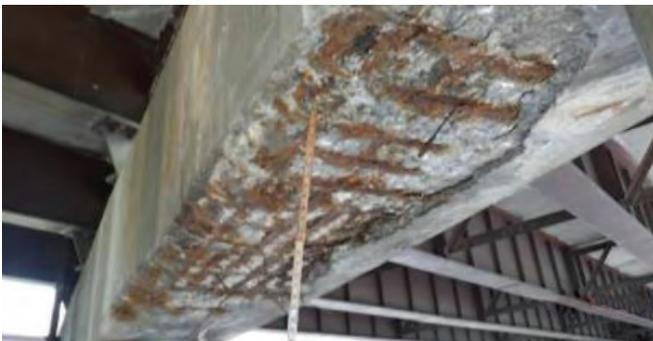
*Extensive pier cap deterioration is just one factor making the I-81 Exit 114 a critical replacement.*
