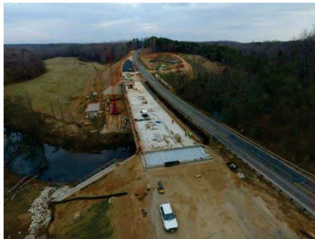
*The existing Route 20 bridge remained in service during construction to maintain traffic and reduce impacts to motorists.*
