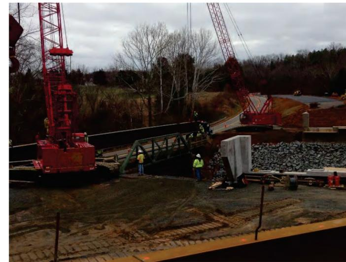
*Steel erection during the construction of the Route 6 bridge replacement*
