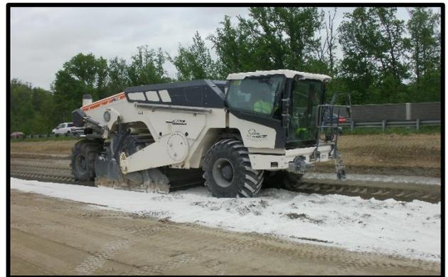
*Soil Stabilization using kiln dust to increase subgrade strength*
