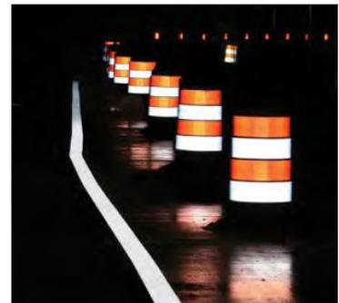
Figure 3.5.3 Wet Reflective Markings Provide Superior Nighttime Visibility
