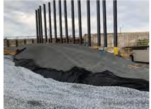
Figure 6 - Lightweight Fill for Bridge Approach
