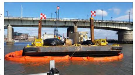
Over-water barge-mounted geotechnical drilling
