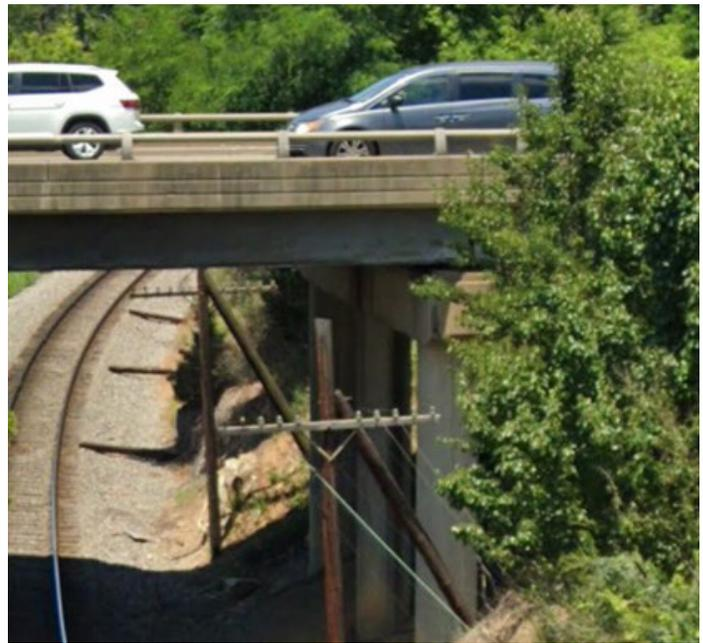
**Figure 5:** Existing Utility Under Bridge and Parallel to Railroad
