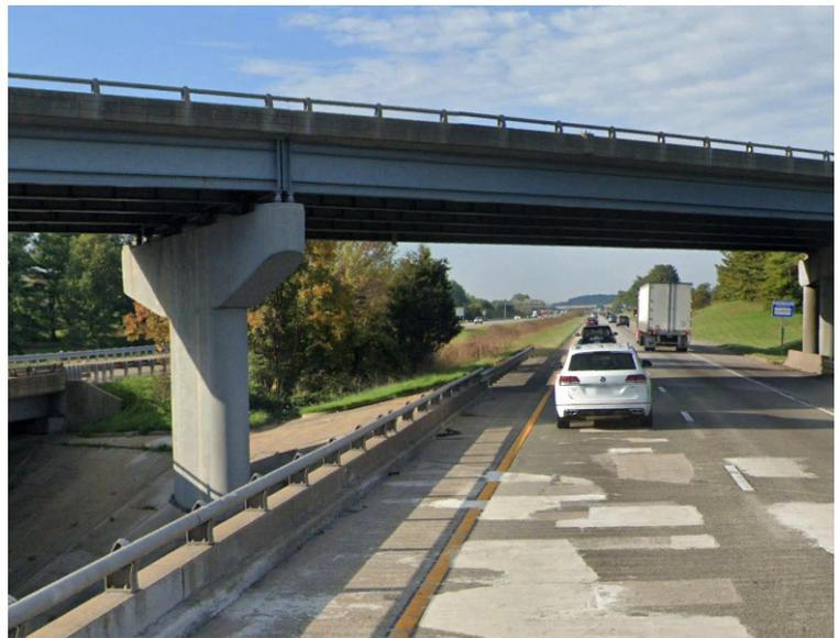
**Figure 4:** Existing Pier Adjacent to Inside Widening
