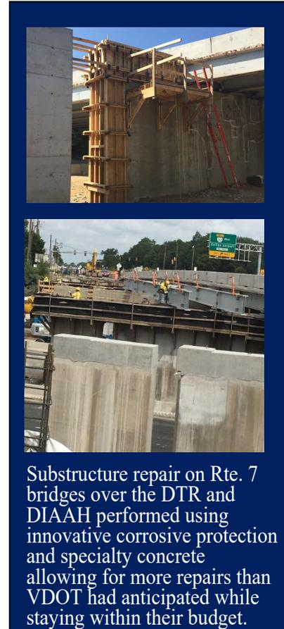
Substructure repair on Rte. 7 bridges over the DTR and DIAAH performed using innovative corrosive protection and specialty concrete allowing for more repairs than VDOT had anticipated while staying within their budget.
