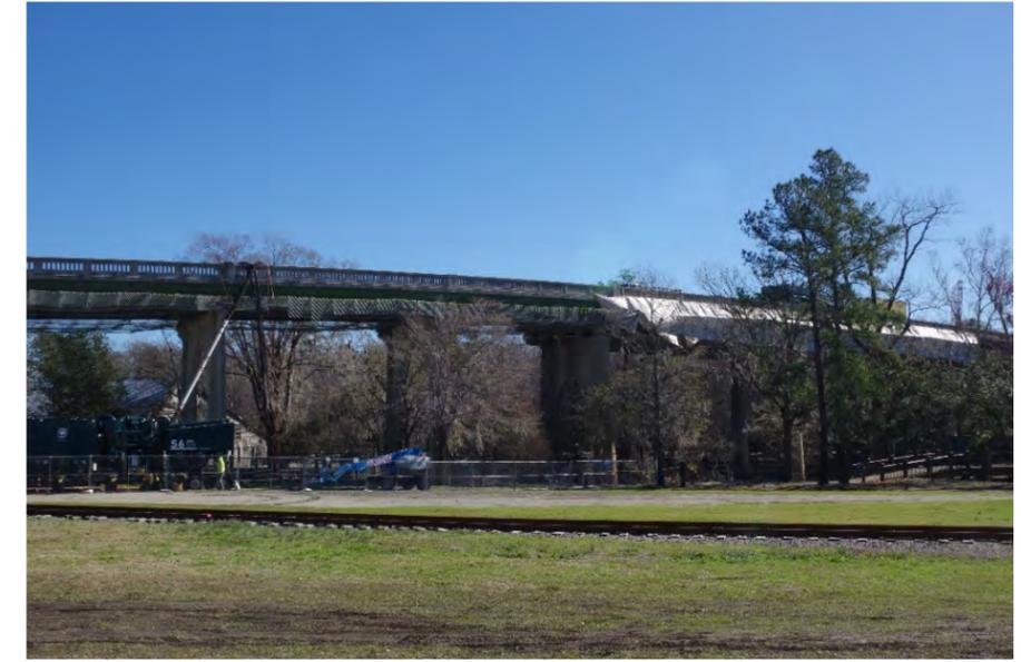
*US 501 Business over Waccamaw River in Conway, South Carolina. Bridge required extensive steel repairs, deck joint sealing, concrete crack sealing, spall repairs and a deck hydrodemolition and overlay.*
