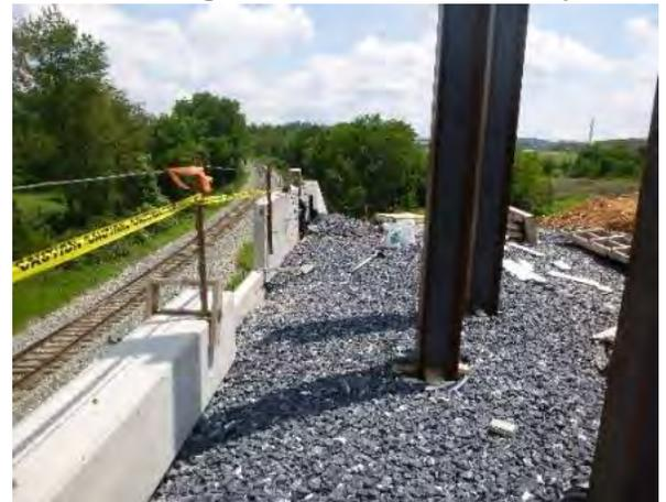
*Figure 4: Pile installed after settlement ceased*
