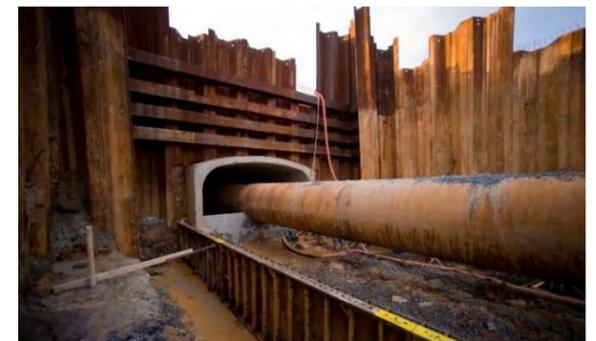
*Shoring for phased culvert reconstruction under I-95*
