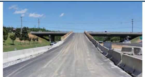
**Innovative Construction Techniques.** A LANE/STV innovative idea involved constructing a median access ramp from a low volume overpass structure to provide construction vehicle access that was SAFELY SEPARATED from highway traffic.
