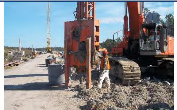
**Geotechnical Mitigation.** Dominion Boulevard’s less severe deeper soils were handled by installing 4,400,000 LF of PV (wick) drains and associated drainage layers. Temporary surcharges were installed to accelerate settlement in these areas.
