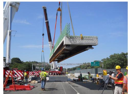
Figure 3.5.4 - Bridge Superstructure Replacement Using Bridge Deck Modules.
