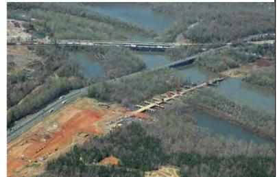
*Construction of the new dual rivers over the Yadkin River using a single temporary construction access work platform.*
