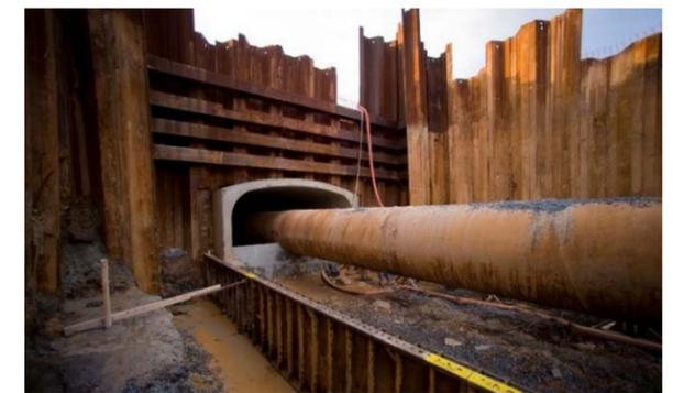
*Shoring for phased culvert reconstruction under I-95*
