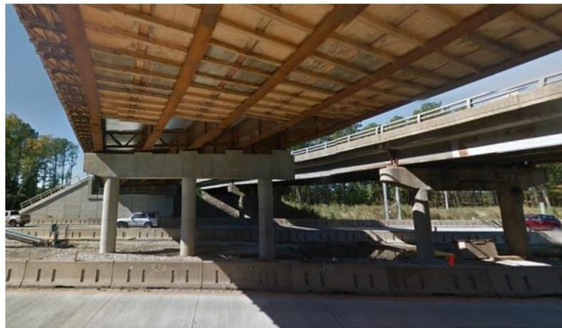
*Staged Construction shown. Old span and new span shown*
