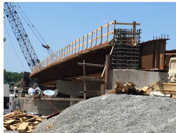
*Two-span steel plate girder with semi-integral abutments*
