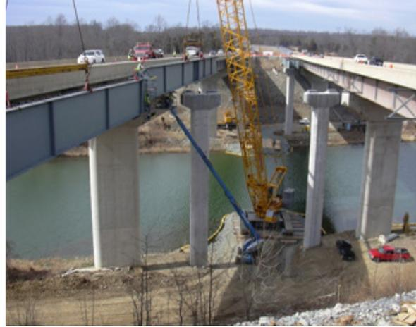
Figure 4 - Constrained Bridge Construction over water.
