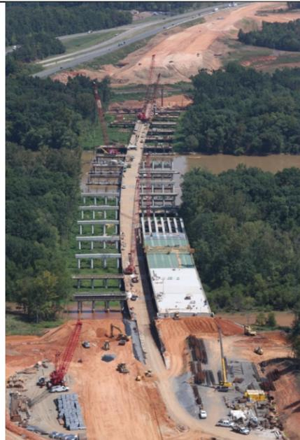
As the lead joint venture partner responsible for construction of this design-build project, Flatiron widened and improved 3.3 miles of I-85 in central North Carolina including new dual mainline bridges (2,900' long) and replacement of the dual US29/70 bridges (800' long) both over the Yadkin River. The scope of work included construction of two additional bridges on I-85 over an active railroad; the removal and reconfiguration of the I-85/US 29/70 interchange; and a new NC 150 Bridge over I-85.
