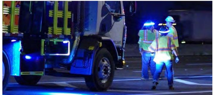
**Figure 3.5-3.** Skanska will explore usage of The Halo Light™, a personal active safety system that attaches to any hard hat and produces a ring of light around the wearer, providing active, 360-degree illumination visible up to ¼ mile away. This offers a distinct advantage in being seen by other personnel, motorists, and heavy equipment operators.
