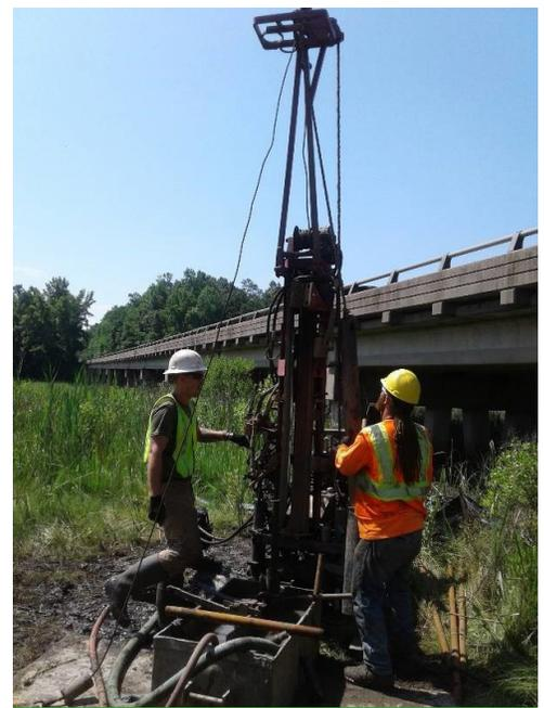
**Smaller drill rig used in wetland area to reduce site disturbance.**
