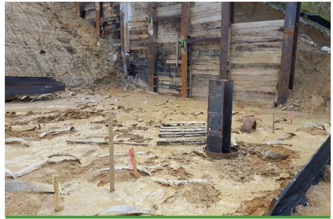
**PVD for pre-consolidation, and pipe piles for slope stability and to reduce negative skin friction - I-64 Segment I.**
