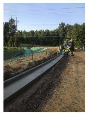
**Photo:** Crews work on the concrete curb and gutter for the approach roadway to Skiffes Creek Bridge.
