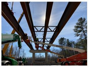
**Photo:** Cranes hold steel bridge beams over Route 143 while crews in bucket lifts secure the beams in place.
