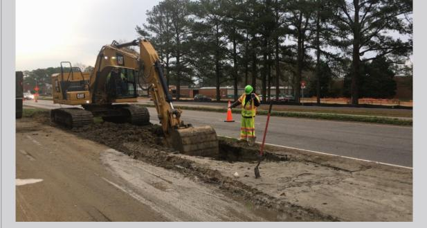
Above: Utility work is a major portion of the Laskin Road Improvements. Over the course of this project, crews will install a total of 3.8 miles of new storm water drainage pipe, 3.1 miles of sanitary sewer pipe and 4.5 miles of domestic water pipe underground. The utility updates are expected to yield significant improvements to storm water management, drainage, and water and sewage systems.
